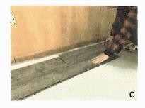
C. Take another long plank, repeat the previous step, insert the long side of plank into long side of previous plank. Then slide plank to your left until the short side is in contact with the short side of the first laid plank.
