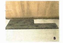
B. The first row must be installed straight. Begin installation back and forth between rows one and two for the first two rows only. Start small plank positioned close to the wall, angle a long plank into the long side of the short plank, and drop long plank tongue into lock. Make sure there are no gaps.
