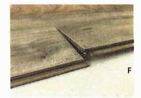
E and F. Finishing rows 1 and 2-- continue alternating planks on rows 1 and 2 to avoid misalignment. From row 3 onwards, installation does not require alternating rows. Install one row after the other by starting with angling on the long side, sliding until the short sides are in contact and then locking the short side. As you go, ensure the short sides are securely locked by tapping with your fist, or if need be, a rubber mallet.
